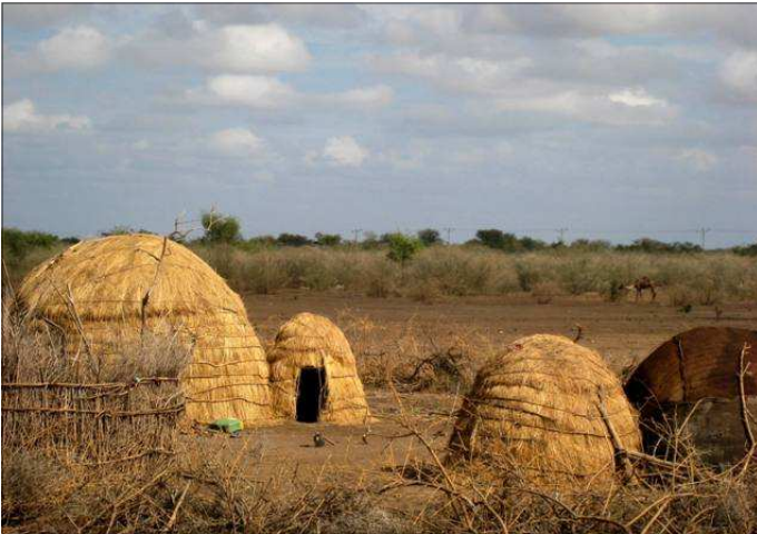
Traditional Afar houses—a lattice framework of sticks covered in thatch, skins and sacking.
